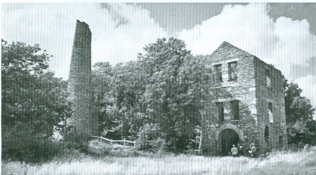
The engine house c.1875 and stack of Holmbush Mine, 19 July 2003.
