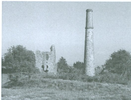
East Kit Hill Mine engine house and stack
