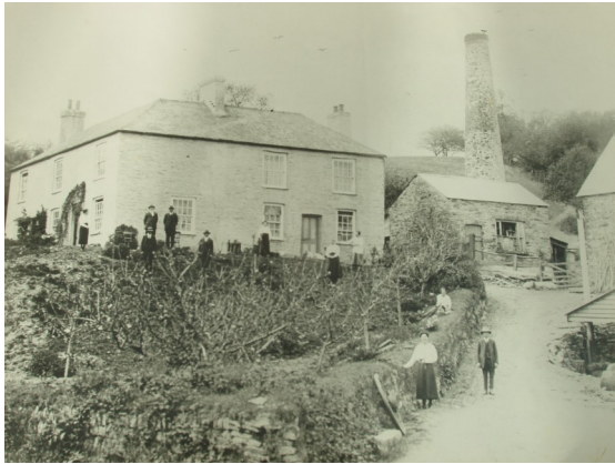
View from the road of East Cornwall Farmhouse c.1910 (left) with the stack and assay house (now garage) (right)
