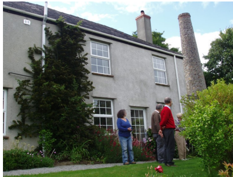
East Cornwall Farmhouse, thought to include the manager's home and couthouse, with the stack associated with smelting and refining processes beyond
