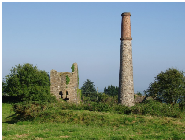
and boiler house at East Kit Hill mine
