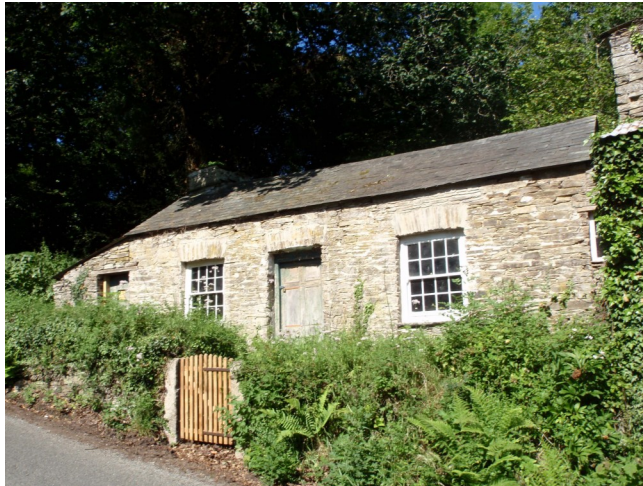
View of the upper cottage looking uphill from the road
