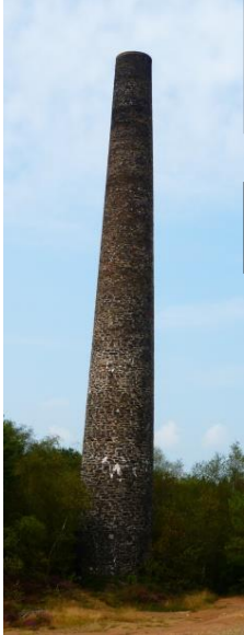
This stack is on the site of earlier ones, but was rebuilt in the 1920s to provide draught for arsenic processing
