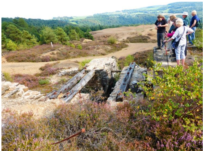
Looking down at the remains of the C19th crusher from the base of the 1850s engine house
