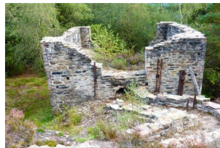
The ruins of the Brunton calciner
