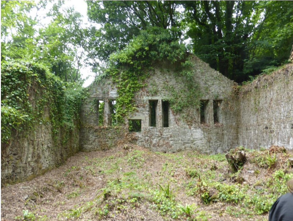
The jigger house with distinctive slit windows
