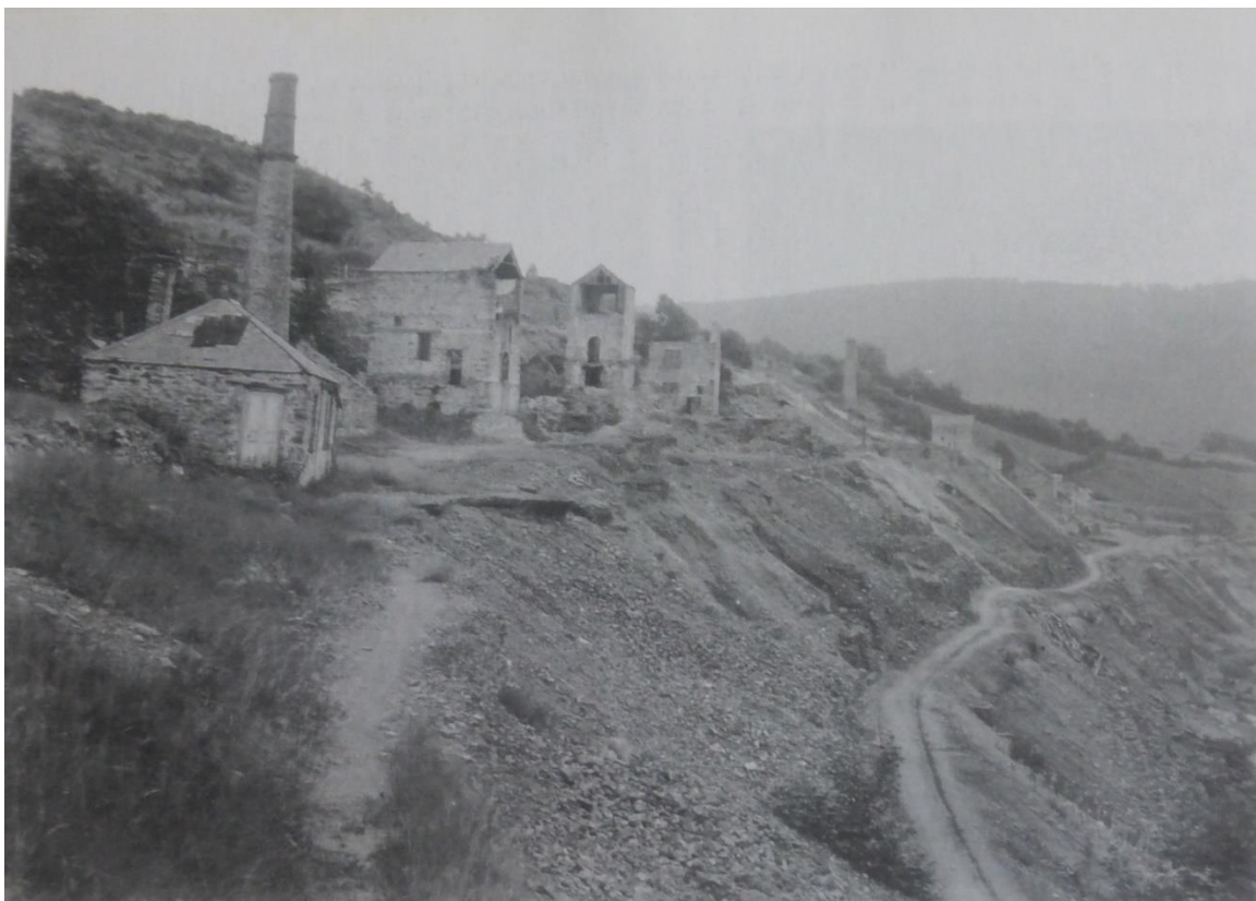
Okel Tor Mine photographed from the west in about 1905. Left to right: count house; part of gable end of dry to right of stack; pumping-engine house; house for winding/crusher engine; crusher house; stamps stack and engine house; gable end of tin plant. (Courtesy John Snell)
