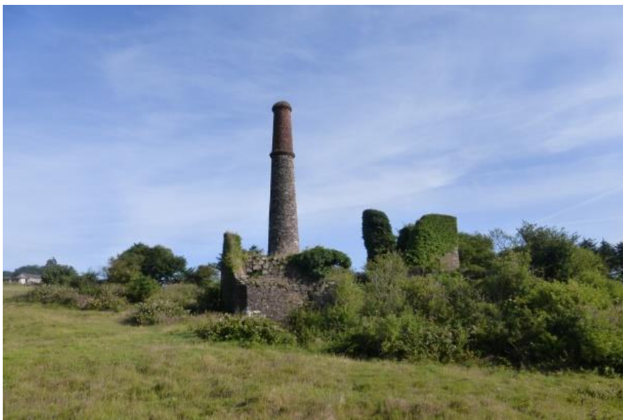
East Kit Hill mine stack, engine house and calciner, July 2015
