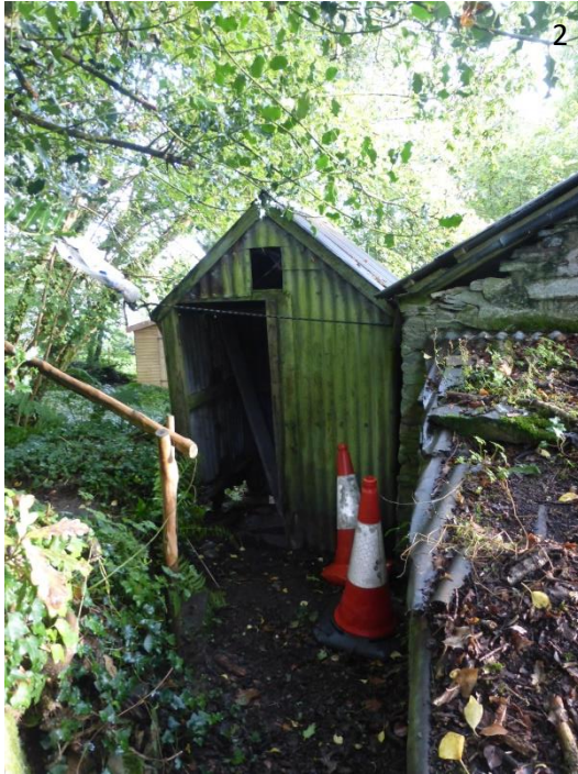
(1) Derwent Dawes checking the privy as it is being winched upright, Spring 2017. (2) As seen on 7 September 2017. The corrugated tin will be restored, a new door fitted, and a seat made to match the original, which has rotted away. Slate floor slabs were revealed after excavation. (3) View of cottages from the cleared garden with Brian Spencer's bench. The bank on the left is the ancient Kerrybullock Park boundary. This shows how the cottages were squeezed in outside the park.
