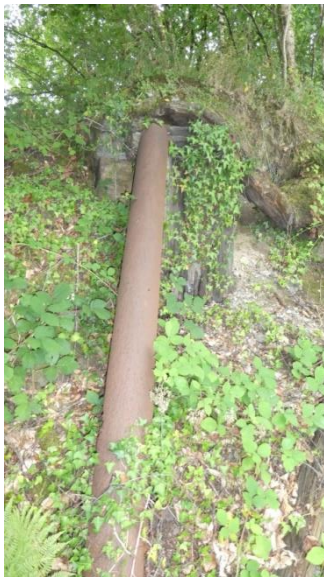
View across the 1st floor of gravity separation tables, largely obscured by vegetation and new tree growth, 14 July 2018
