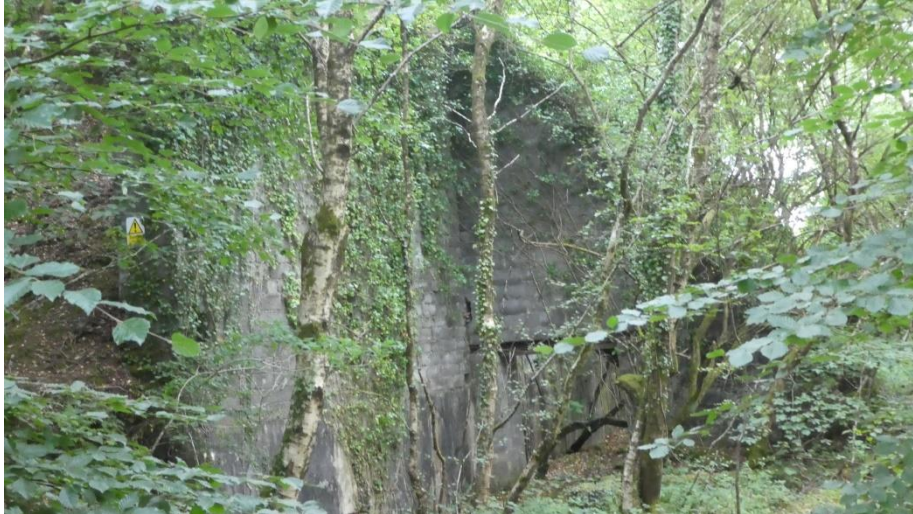
The support of the aerial ropeway, 14 July 2018
