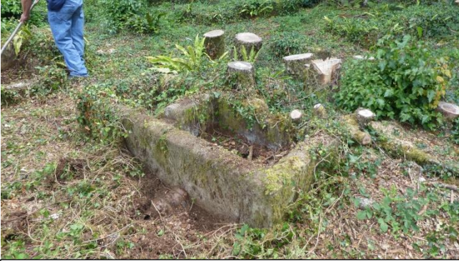
right: The back retaining wall, with pipe exits two-thirds of the way up along its length. At the centre a buttress-like channel bringing water from above, with oblong outlet at the bottom. Lined up with the 'buttress' and in the foreground with ferns were two deep slots, 14 July 2018
