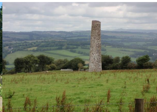
Stack from arsenic flue of Luckett Mine above Deer Park Farm, Luckett, 2012, replacing earlier one lower downhill
