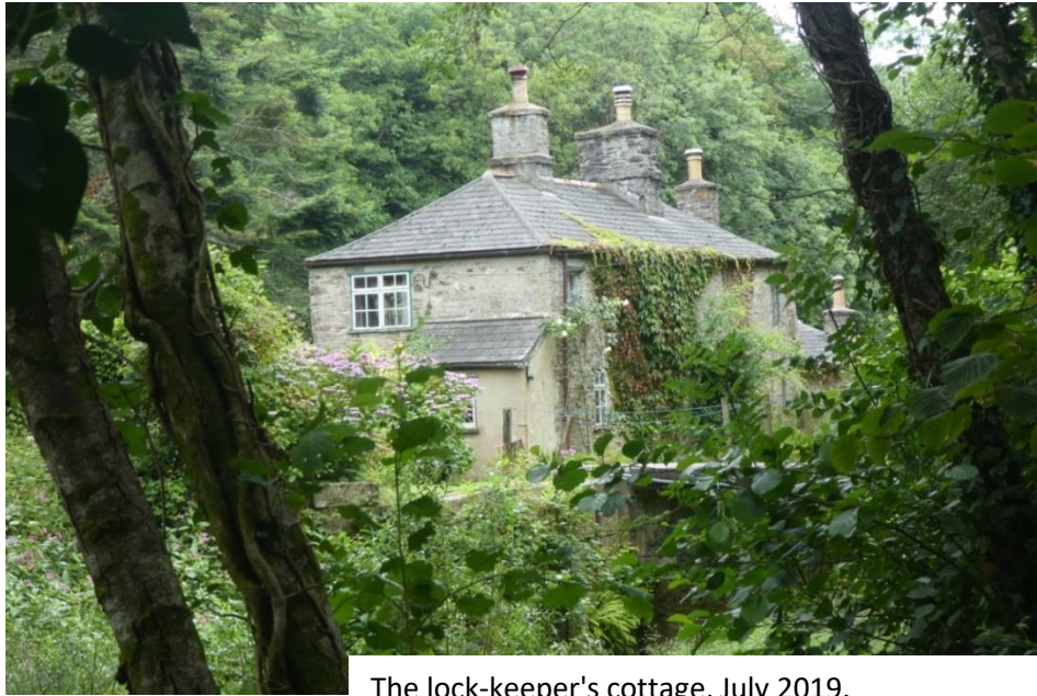
The lock-keeper's cottage, July 2019.
