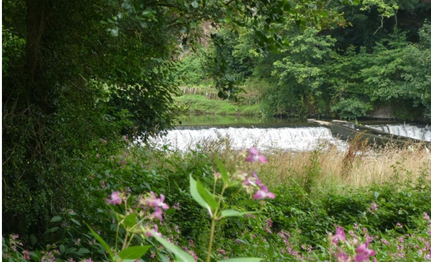
The modern weir with salmon-leap in centre, July 2019.
