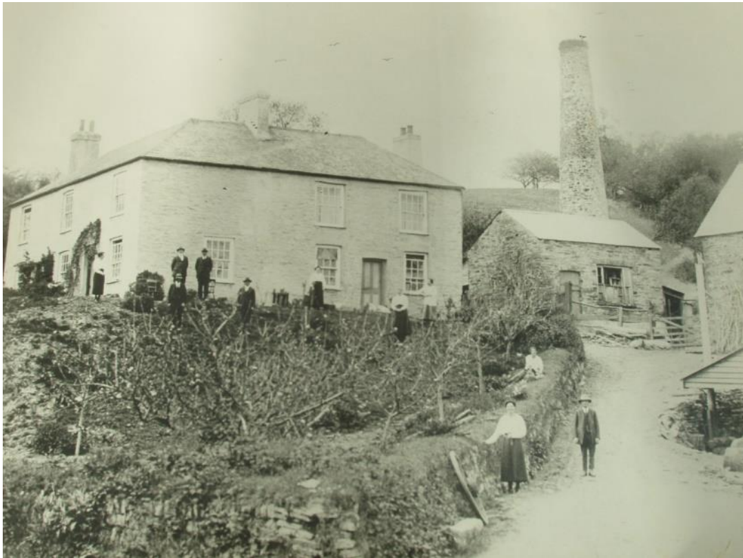
East Cornwall Farmhouse, Harrowbarrow , from the road c.1910, with stack and assay house. Lead and silver were mined here (1810-1880s), and unusually were also smelted and refined on site.
