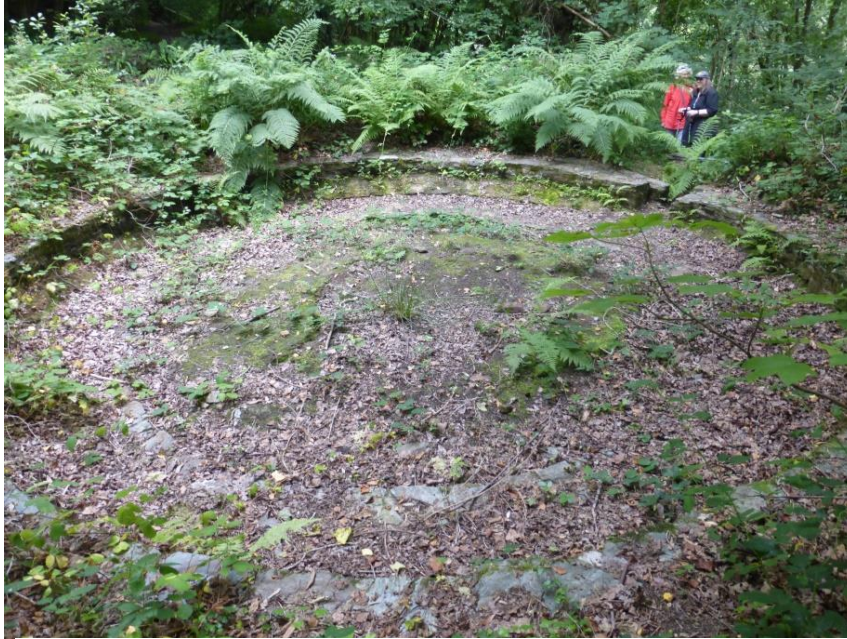
One of 4 round buddles used in the dressing of tin process at Okel Tor, Calstock , July 2016. Hosted by Nick Cole.
