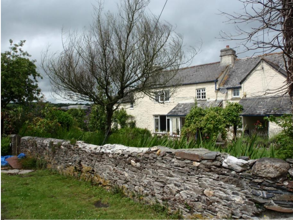
North Hooe Farmhouse, Bere Alston , visited during an excursion into Devon, courtesy of Penny Rowe, July 2011.
