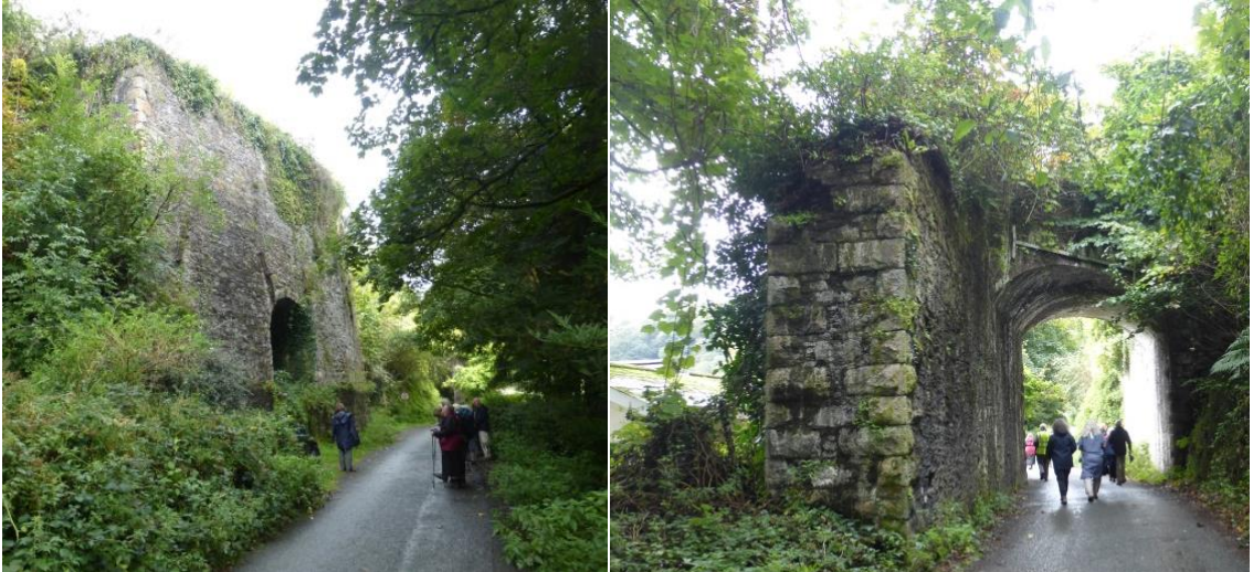
Calstock Quays , September 2017. Lime kiln incorporated into incline railway support & incline railway bridging the road. Most lime kilns date from 1770-1830, lime was roasted in kilns to be spread on fields to counter acid soil.
