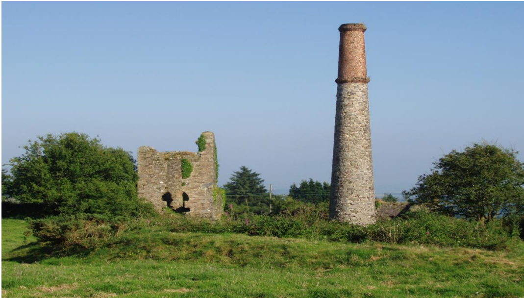
The boiler house and stack at East Kit Hill Mine, July 2011. In 2009 a lightning conductor was fitted to the stack. The work showed that there were two tunnels linking the boilers to the stack. One had been blocked as it was superseded by the second required after the boilers had been enlarged.
