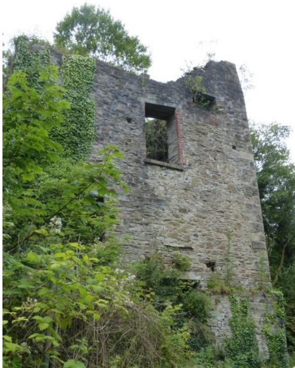
Whim engine house, Gunnislake Clitters Mine , July 2015. This structure held a 24-inch beam whim engine to wind ore up the shaft and to power the small copper crusher. The mine closed in 1889.
