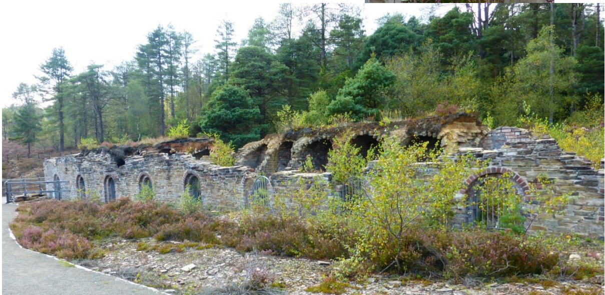
Another trip into Devon to Devon Great Consols , September 2014. The 1920s arsenic condensing chambers provide an iconic image. Arsenic bearing rock could be refined into 99% pure arsenic.
